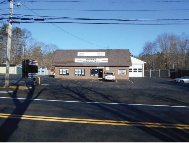
Front View Building 3 Midway Auto Parts
