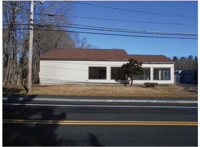
Front View Building 1 Former Garden Equipment
