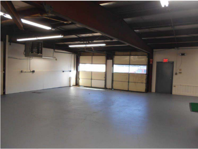
Building 1 Interior Rear Area
