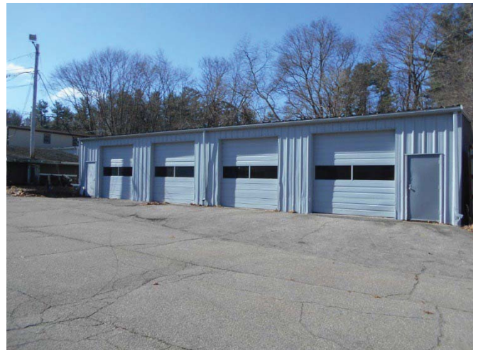
Front View Building 2
