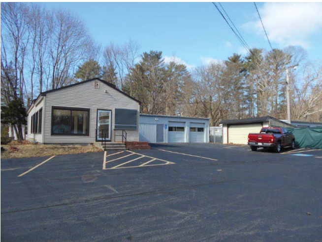
Side View Building 1 Former Garden Equipment
